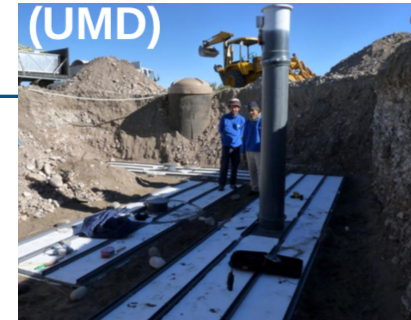
(UMD = Underground Muon Detector)
